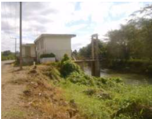
Water Intake Pump House on Waimanu River
