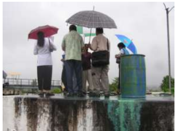
Copper Sulphate dosing at Flash Chamber
