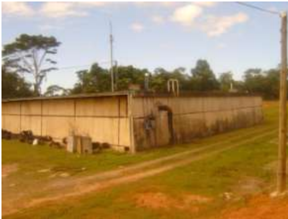
Raralevu Reservoir – Concrete
