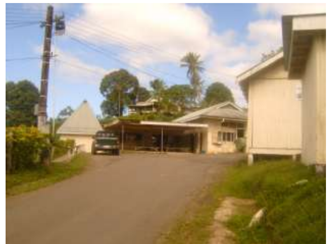
Rewa Water Supply -Office
