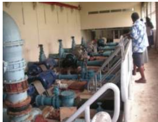
Electrical uplift pumps – Waila Plant
