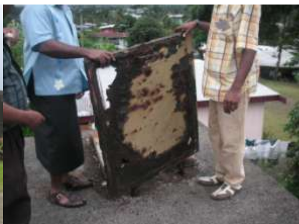
Reservoir inlet lids are rusted and unplaced
