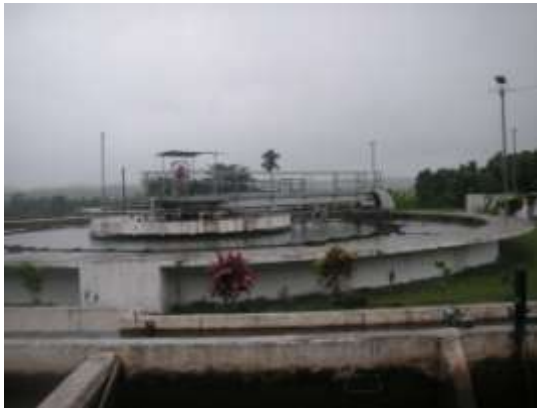
Clarifier – Waila Plant
