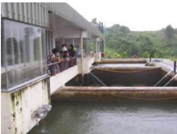
Rapid Sand Filters being cleaned – backwash
