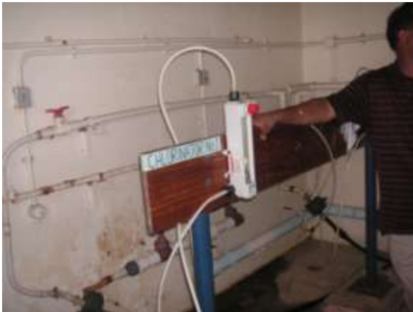
Functioning Chlorinator –Waila
