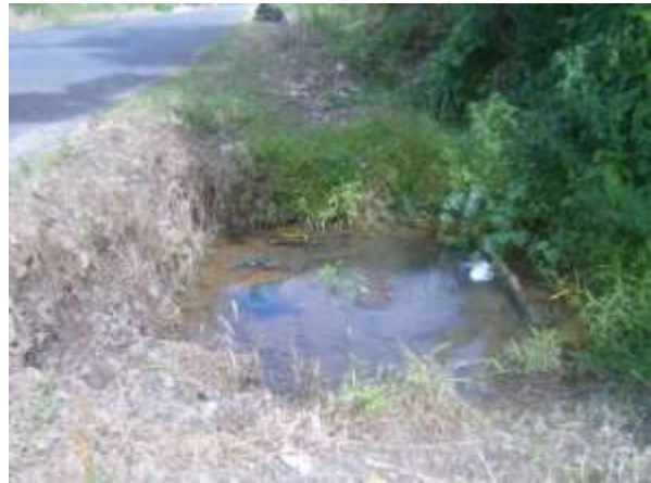
Leaking Mains Keys – Rewa Delta
