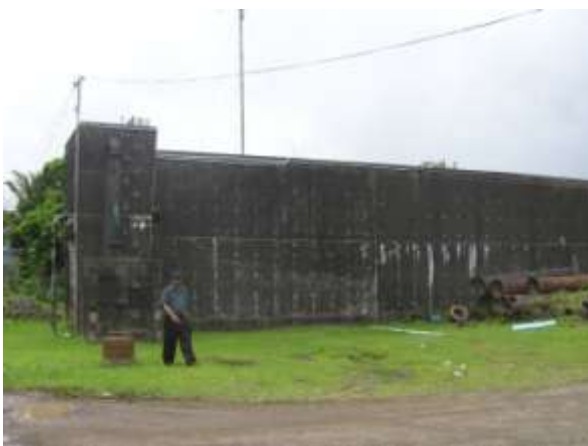
Concrete Reservoir- Kalabo
