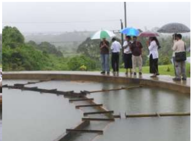
One of the three clarifiers – Waiala Plant
