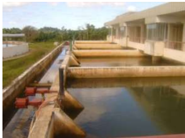
Rapid sand filters- Waila Plant
